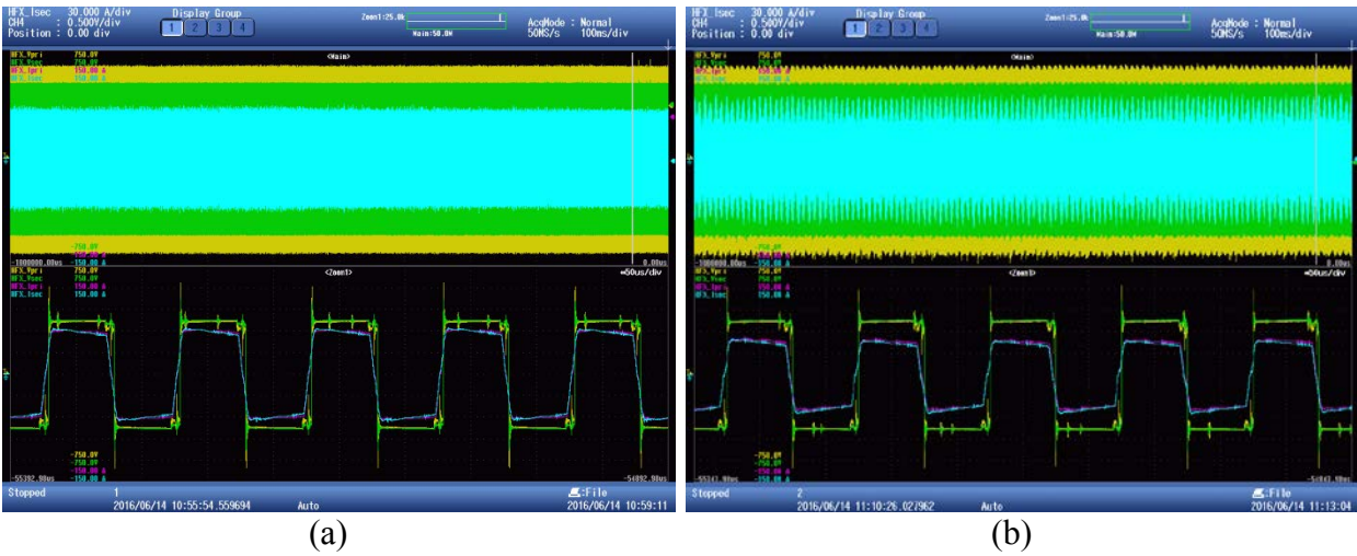
Figure 10. CUBE in Battery-Only mode and high proportional gain for 0-component of FLI voltage control PID feedback loop, DAB waveforms at (a) 21-kW balanced load and (b) unbalanced load of PhA = 12 kW, PhB = 6 kW, and PhC = 3 kW.
