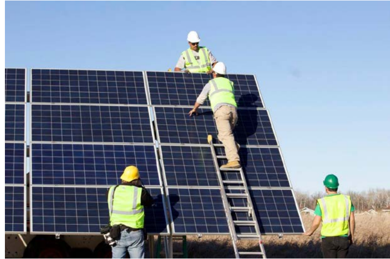
Installing one of the five solar PV projects
