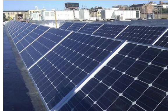
30-kW rooftop PV array that powers the Forest County Potawatomi Community administration building
