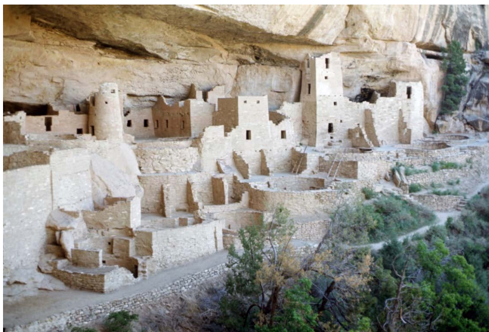
Figure 1. Thoughtful home designs on tribal lands have long provided shelter adapted to regional climates. The Anasazi Cliff Dwellings were built into depressions in cliffs providing shelter and comfort across seasons.
