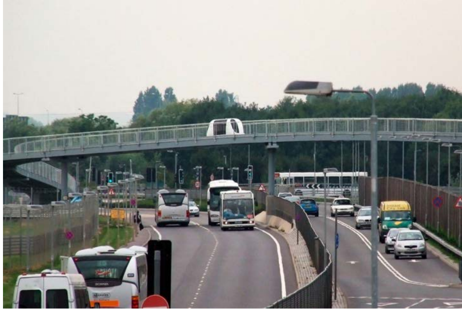
Figure 10. Lightweight infrastructure for the London Heathrow International Airport small four-passenger vehicle system.
