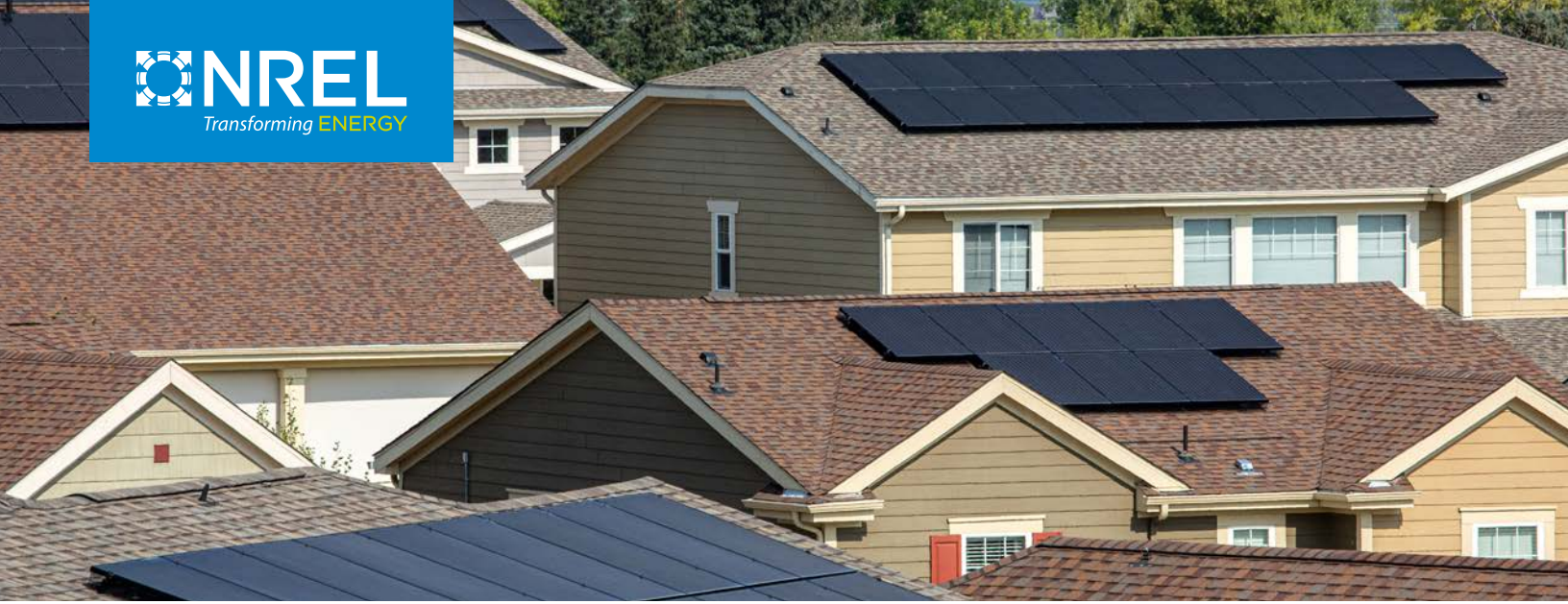
Photo by Werner Slocum, NREL 66353
