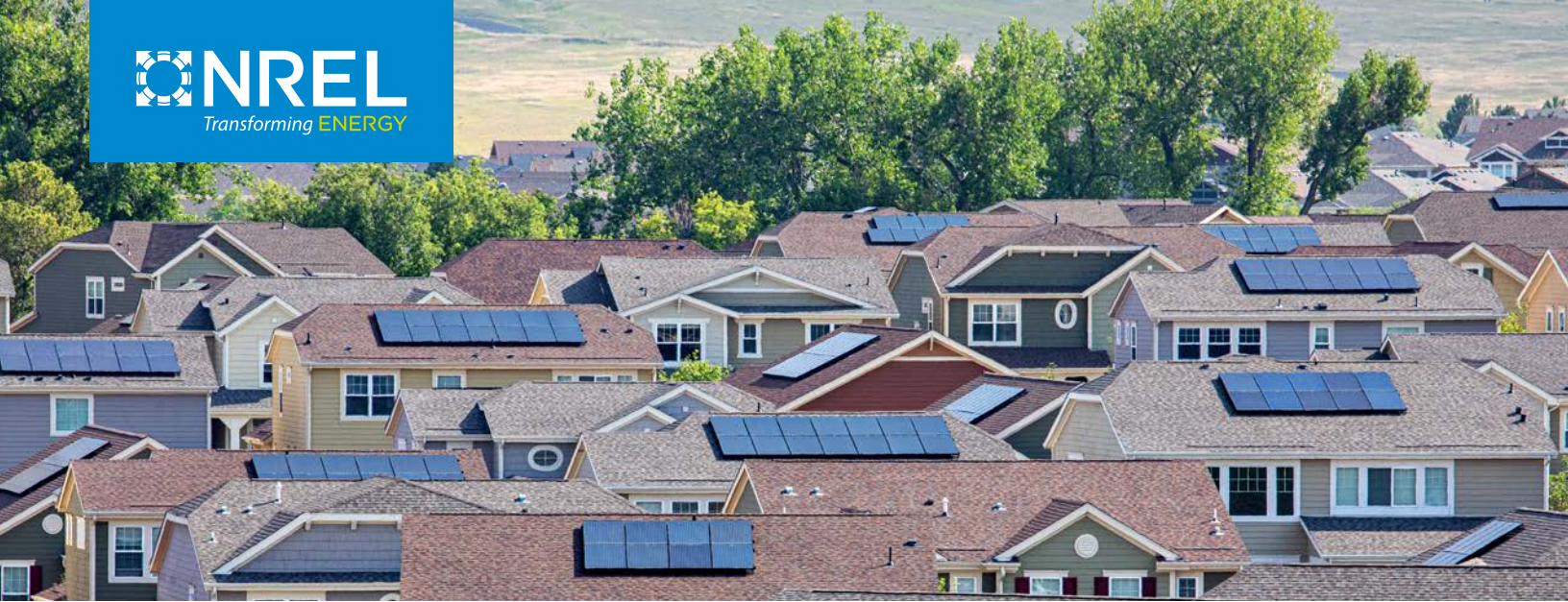
Photo by Werner Slocum, NREL 66338
