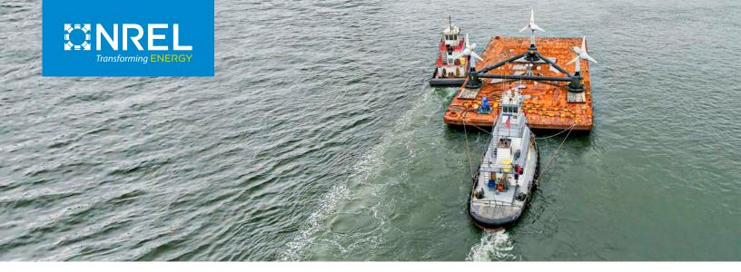
Verdant Power successfully installed an array of tidal turbines at the Roosevelt Island Tidal Energy Project in New York City's East River. Photo from Paul Komosinski, Verdant Power.
