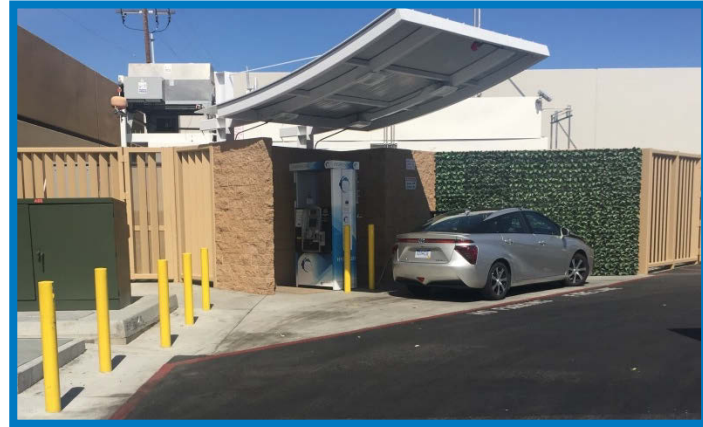
Air Liquide, Anaheim, CA. Photo: NREL
