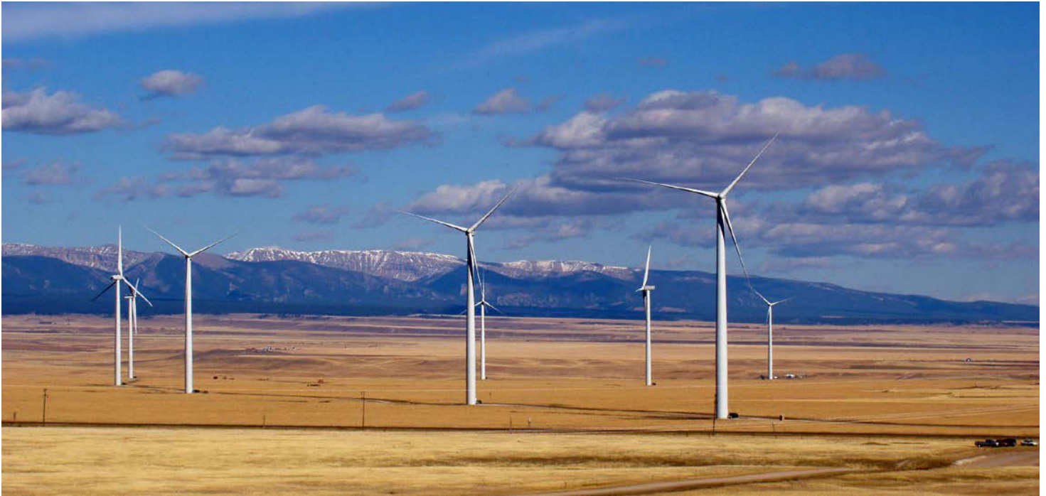
Judith Gap Wind Energy Center, Judith Gap, Montana 135 MW, 90 GE 1.5 MW SLE turbines Photo Credit: Mark Jacobson
