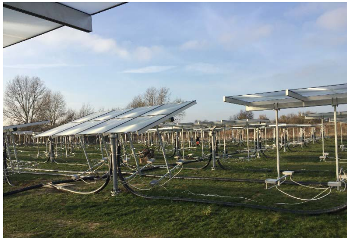
Figure 40. Heliac 2-MW th demonstration for a district heat facility in Denmark. Photo provided by Heliac, credit Heliac.
