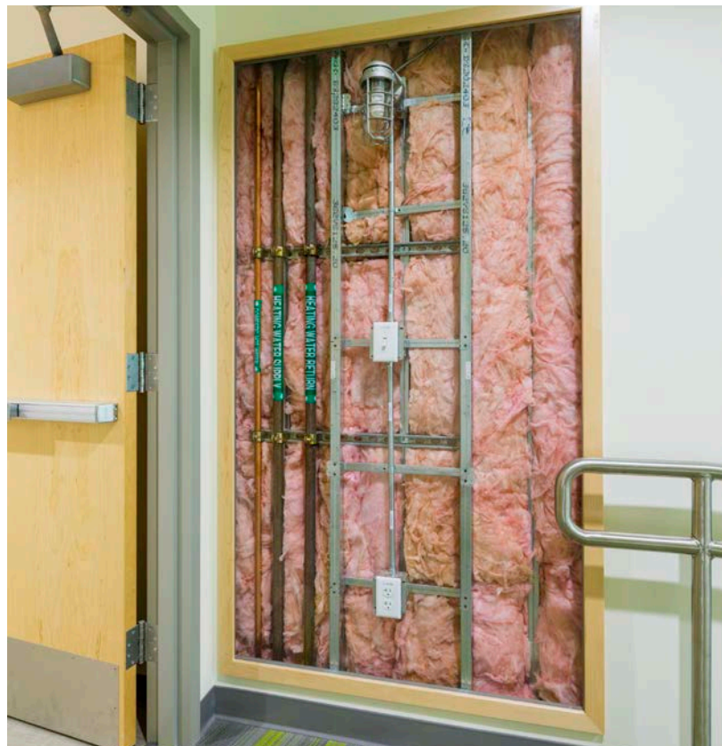
See-through building sections, like this "truth wall" at Emerald Elementary School in Broomfield, Colorado. Designed by RB+B Architects and Fielding Nair International, Photo by Paul Brokering Photography
