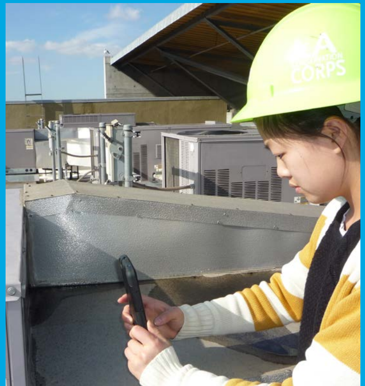
After learning about safety and security, Student Energy Auditor Training program students at LAUSD spend time inspecting HVAC systems and learning how to review and collect data. Photo by LAUSD
