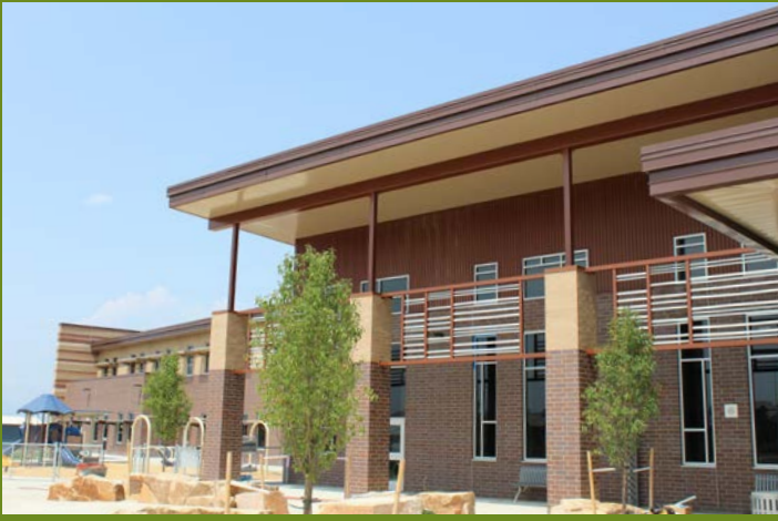
The Thunder Vista P-8 EUI target is 26kBtu/ft 2 -yr, the lowest in the district. Photo by Paul Torcellini, NREL
