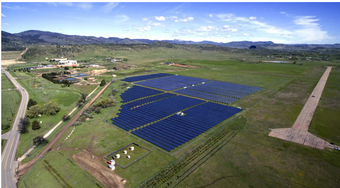
Figure 4. 5.3 MW solar PV array at Christman Field on CSU's Foothills Campus
