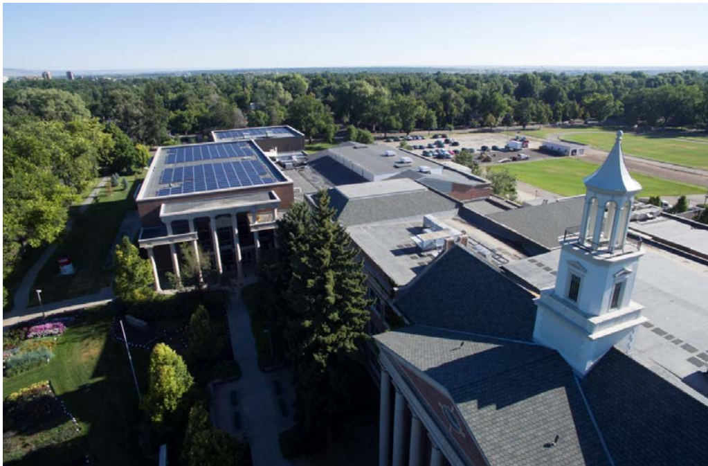
Figure 6. Rooftop PV on CSU's University Center for the Arts
