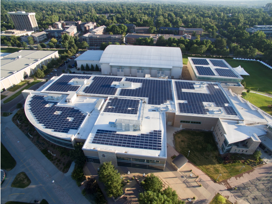
Figure 5. Rooftop PV on CSU's Student Recreation Center
