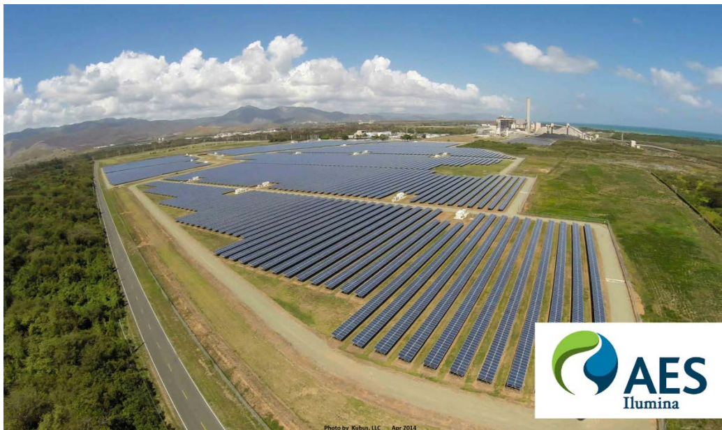
Figure 14. Aerial view of the Ilumina PV power plant. Image from AES
