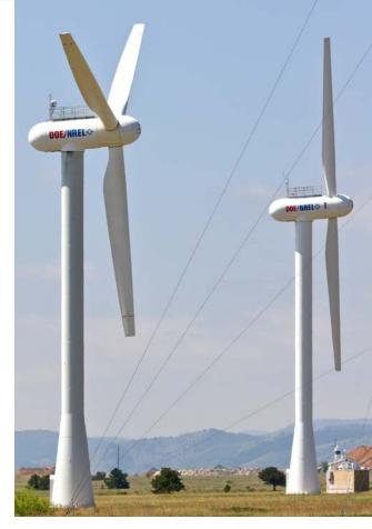
The NWTC's experimental wind turbines, a three-bladed Controls Advanced Research Turbine (CART3) and a two-bladed CART2. Both are used to validate new control schemes and equipment for reducing loads on wind turbine components. *Photo by Lee Jay Fingersh, NREL 21664*
