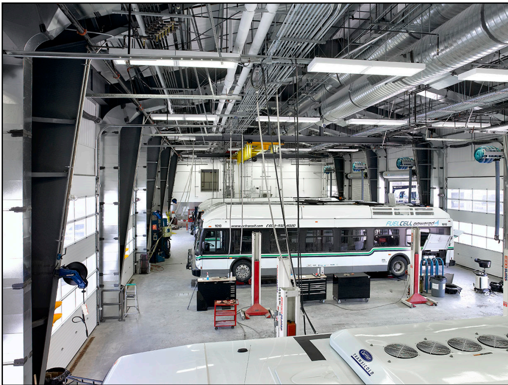
Figure 7. Maintenance facility. Photo courtesy of BC Transit
