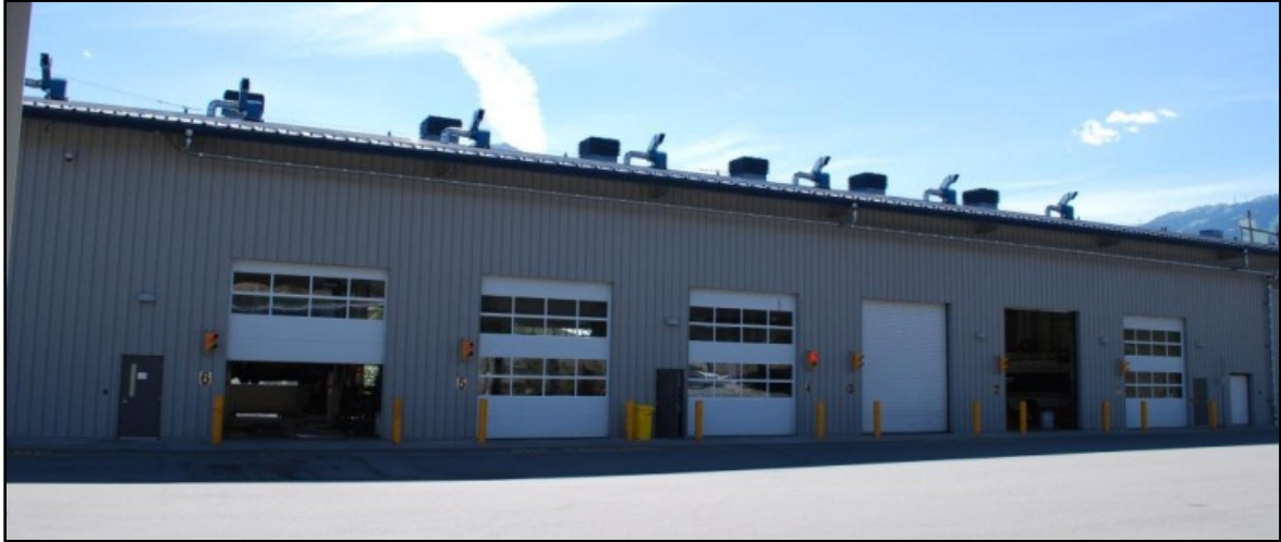
Figure 6. Whistler Transit maintenance facility
