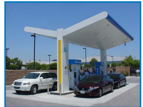
APC/Shell Pipeline station, Torrance, CA. Photo: NREL
