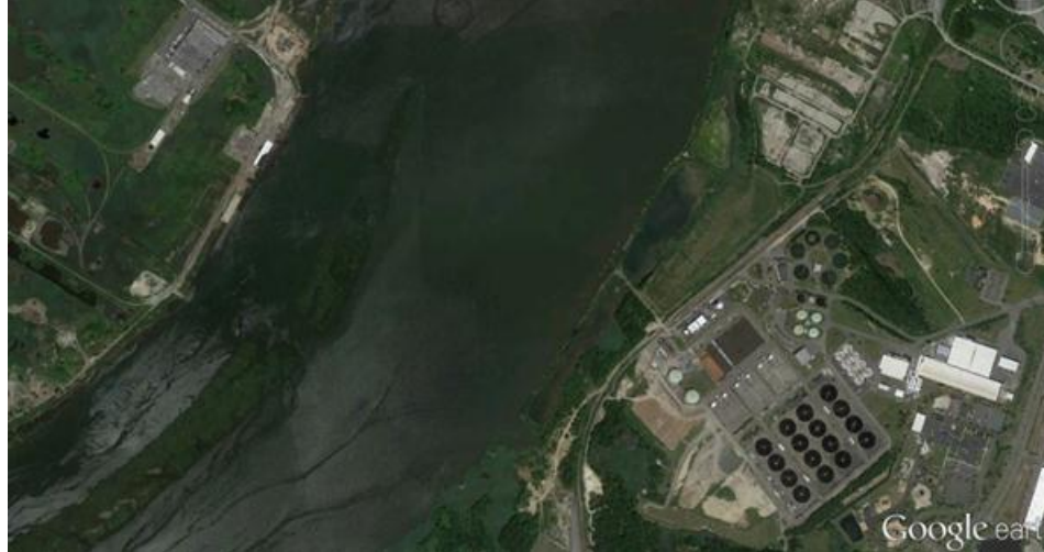
Figure 17. Middlesex County Utilities Authority Wastewater treatment facility in Sayreville, New Jersey
