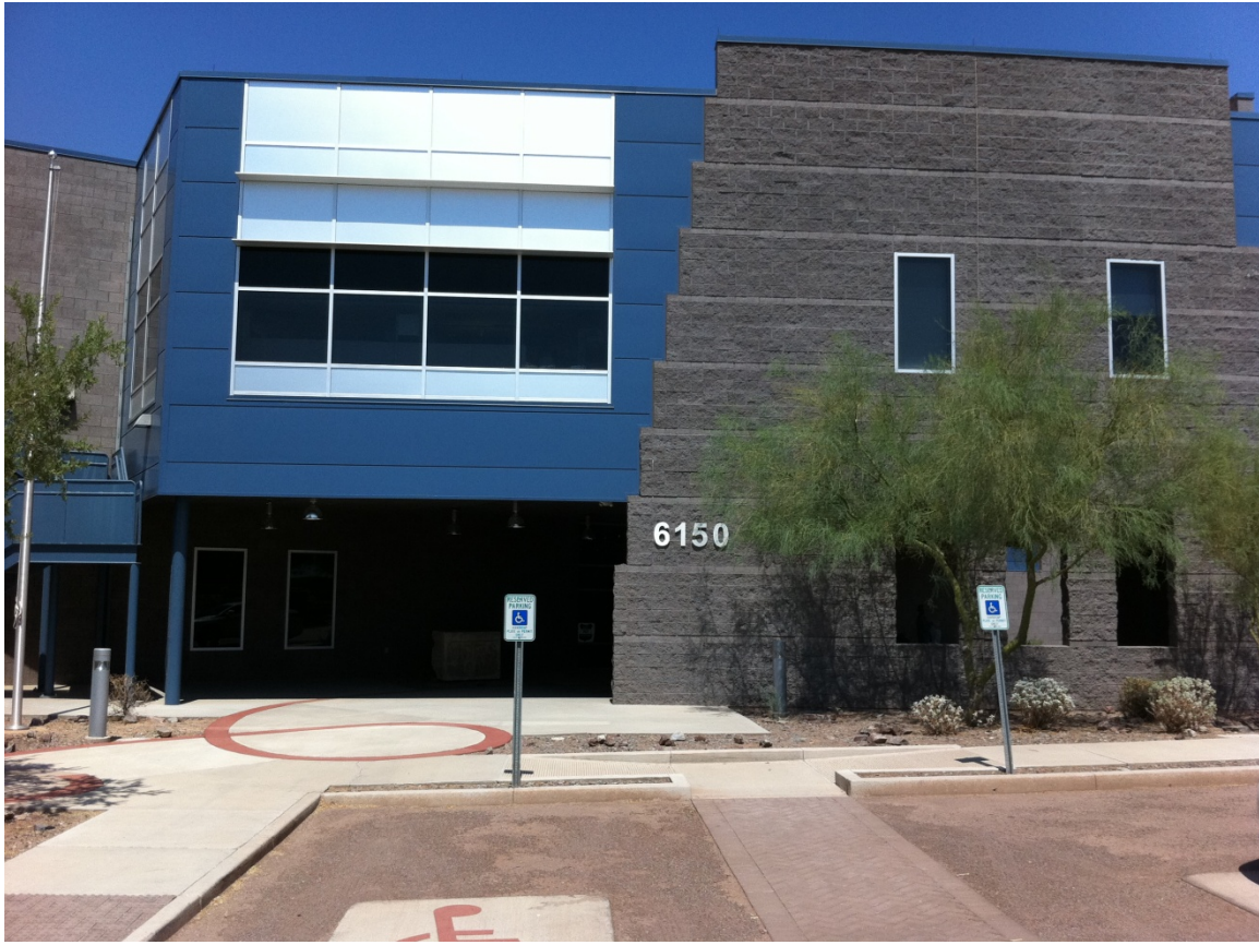
Figure 5-2. Phoenix Area Office south elevation view. Photo by Otto VanGeet, NREL
