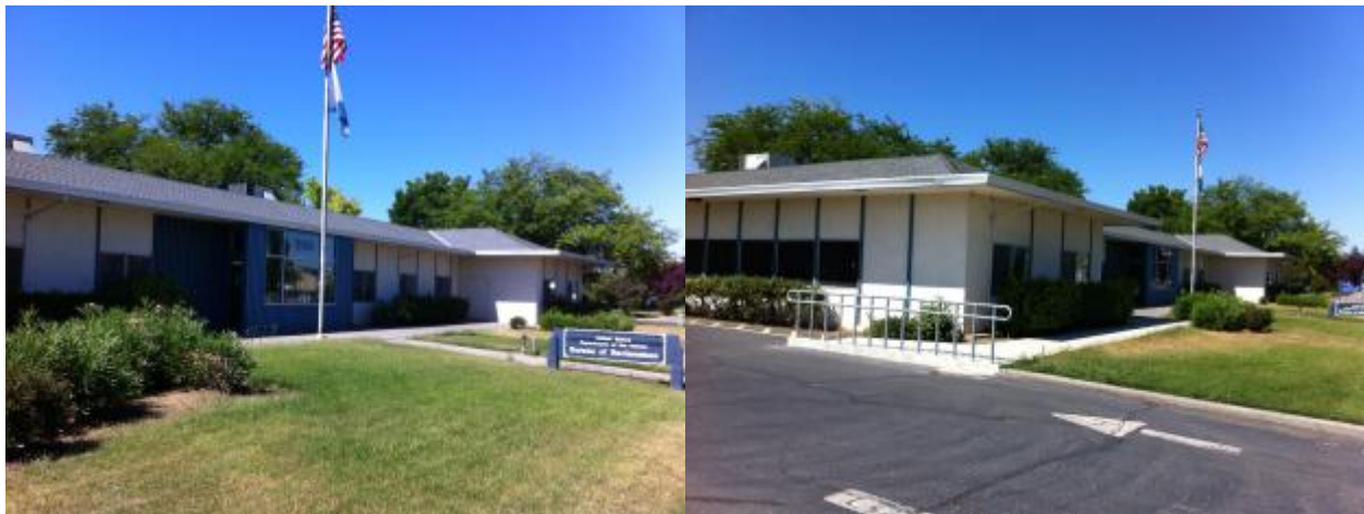
Figure 6-2. Willows Office entrance and north elevation view (left), and Willows Office northeast view (right). Photos by Otto VanGeet, NREL
