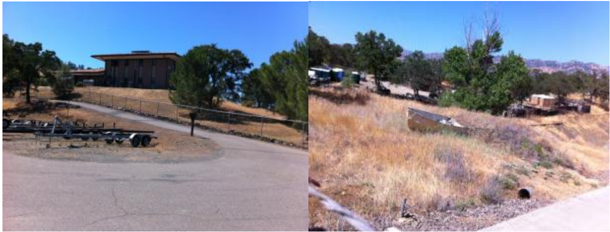
Figure 6-15. PV Area 2 beyond fence looking north (left) and PV Area 3 looking northeast (right). Photos by Otto VanGeet, NREL
