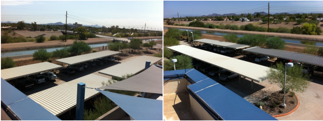
Figure 5-11. Existing carports looking southeast (left) and looking northeast (note existing PV on east-most carports) (right). Photos by Otto VanGeet, NREL
