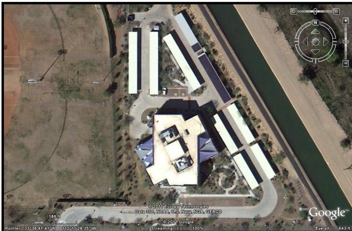
Figure 5-1. Aerial view of Phoenix Area Office
