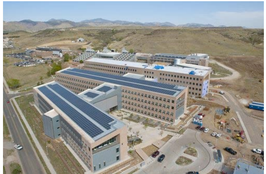
Photo by Dennis Schroeder, NREL/PIX 19089
