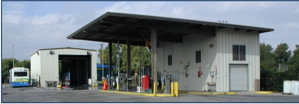
Figure D-2. CNG fueling lane and bus wash (Thousand Palms)
