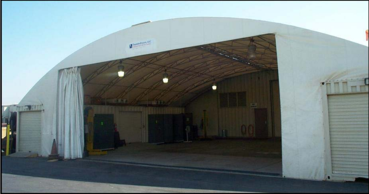
Figure D-7. CNG maintenance facility in Thousand Palms (top) and hydrogen maintenance building (bottom)
