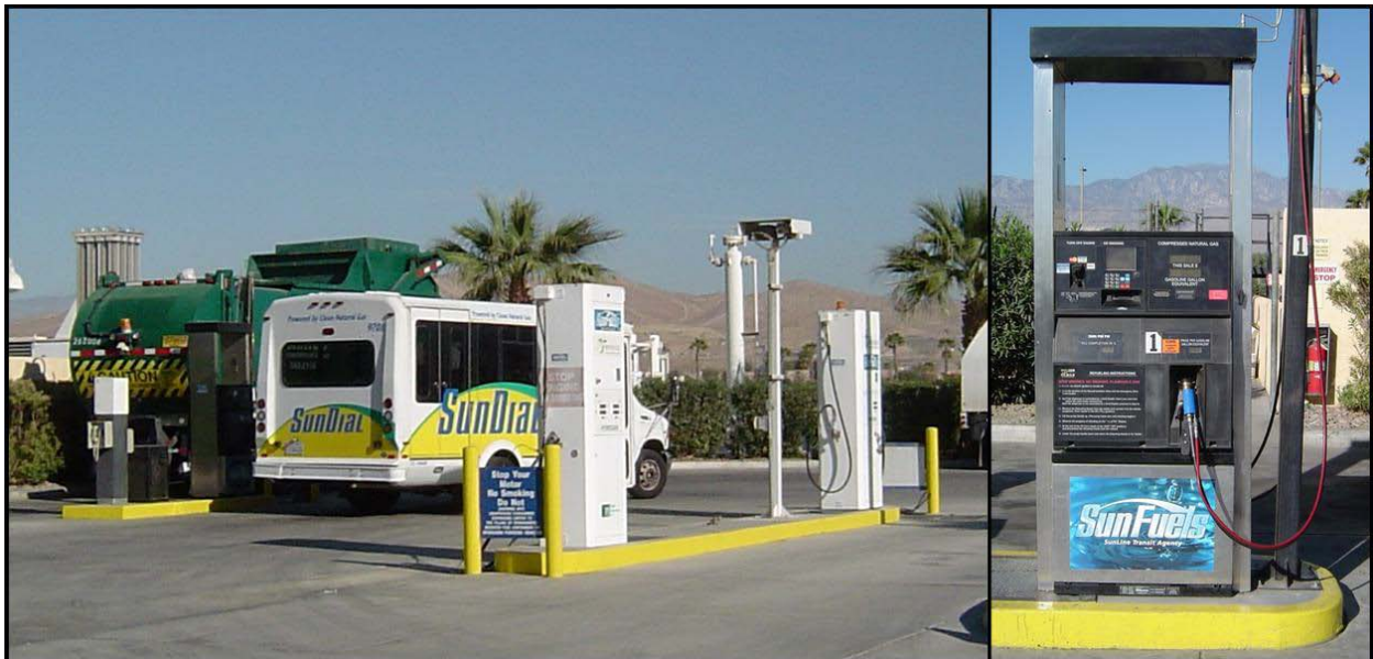
Figure D-1. Public fueling at SunLine's Thousand Palms CNG fueling station
