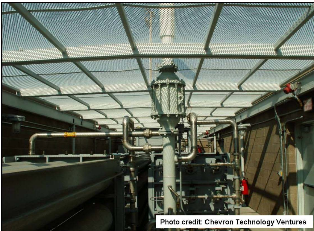
Figure D-3. Cascade hydrogen storage vessels at AC Transit station
