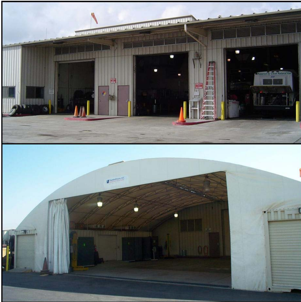
Figure C-8. CNG maintenance facility in Thousand Palms (top) and hydrogen maintenance building (bottom)
