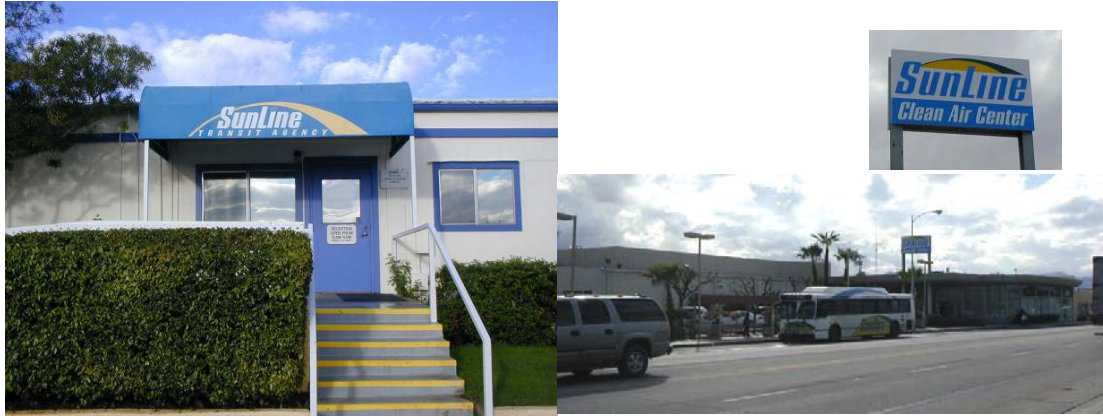
Figure A-2. SunLine headquarters in Thousand Palms (left) and Indio bus garage (right)
