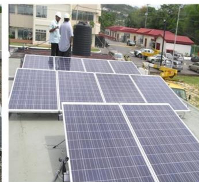
Trinidad and Tobago Electricity Commission Mt. Hope Compound (2.2 kW)
