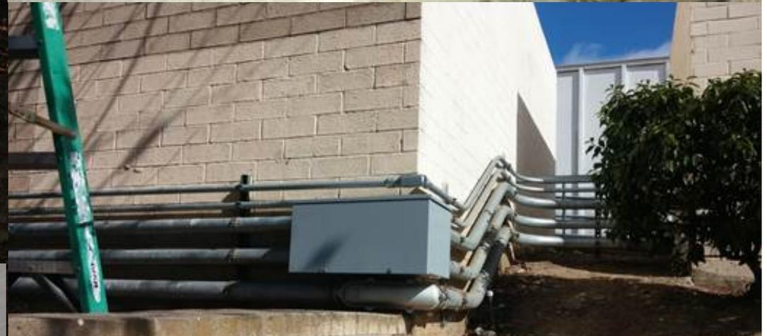
**The Fix:** A box replaces LB fittings and new cables are installed. I consider this a partial fix because LB fittings are still present -- those runs probably passed the megger test...
