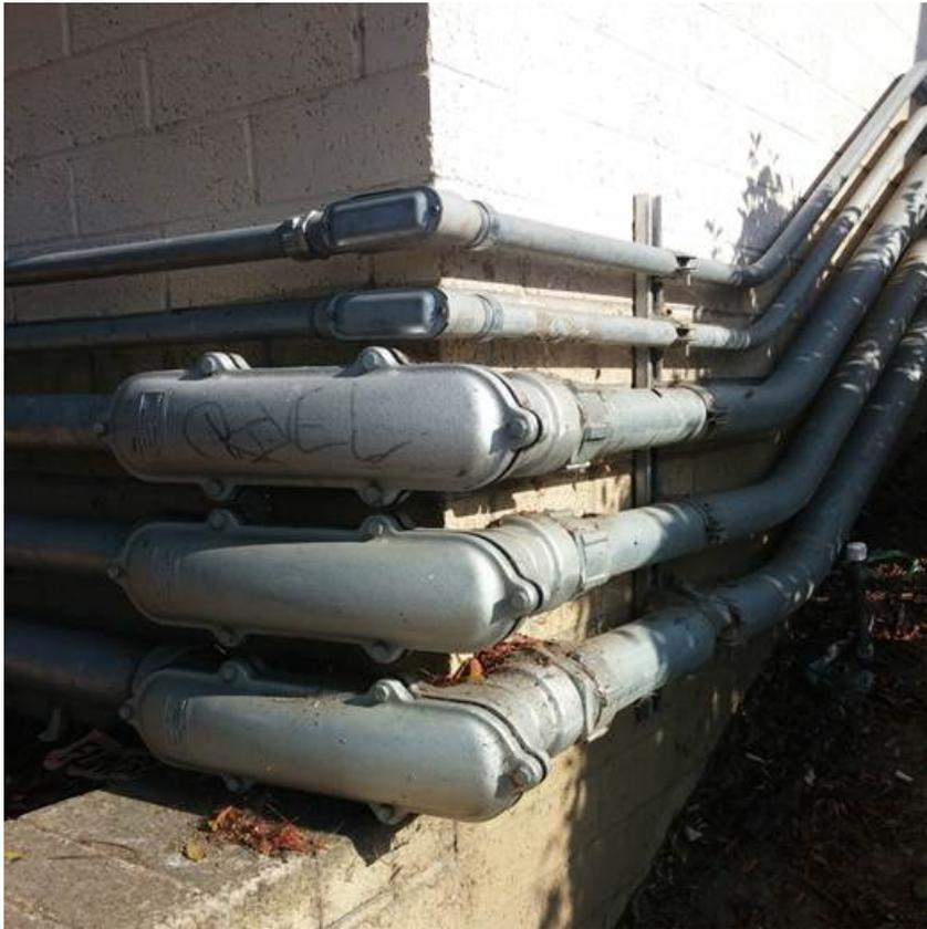
**The Scenario:** LB fittings run DC outside a building. Probably built circa 2007-9. Failed megger test last year.
