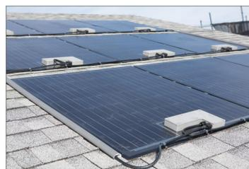
Glass-less modules attached using an adhesive approach
