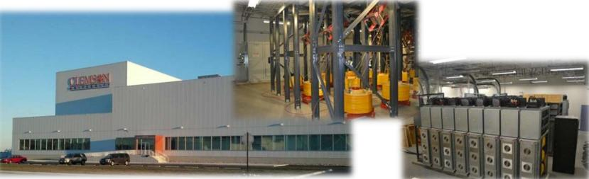
"eGRID is a utility-scale electric power laboratory combining real time grid simulation capabilities with a highly configurable, multimegawatt, medium voltage three phase experimental grid."
