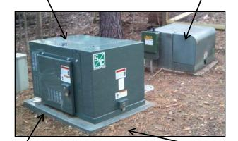
**Battery vault** 4-feet deep, open bottom **Battery (underground in vault)** 25 kW / 25 kWh Kokam Li-ion battery pack
