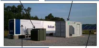
**Battery container** 750 kWh/250 kW Lithium Polymer Includes Batt. Mgt. System
