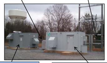
**Battery container** 402 kW/282 kWh NaNiCl batteries (12 cells) Inverter/Controls Storage Management System (SMS) 1.25 MVA capacity/1.0 MVAR capacity
