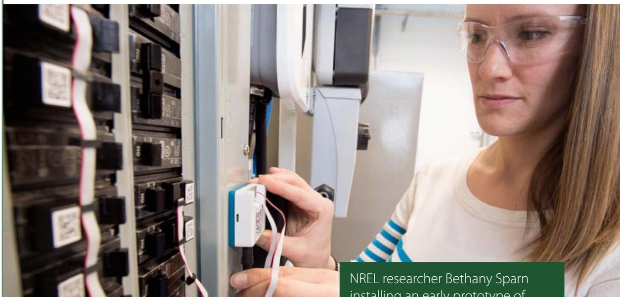
NREL researcher Bethany Sparn installing an early prototype of the Whisker Labs technology in NREL's Energy Systems Integration Facility's Systems Performance Lab. Photo by Dennis Schroeder/NREL
