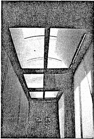
Fig. 12. Movable insulation system for skylights, Daxing.
