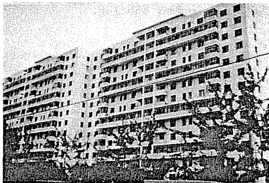
Fig. 4. New apartment construction in Beijing showing the south side.
