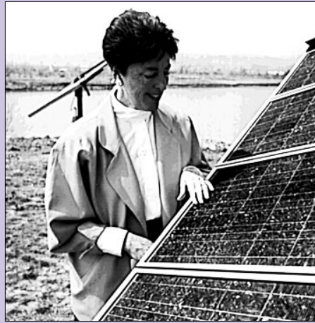
Mayor Susan Thornton examines one of 40 solar panels providing clean, renewable electricity to a park irrigation project in Littleton, Colorado.
