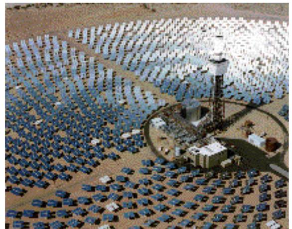
**Power tower technology—**To improve power tower (central receiver) technologies, SunLab and Rockwell International are developing an advanced receiver that is smaller and more efficient than current designs. Researchers also are working with several utilities to examine the feasibility of building hybrid power towers that run on both solar energy and natural gas. Hybrid power towers run continuously throughout the day and night.
