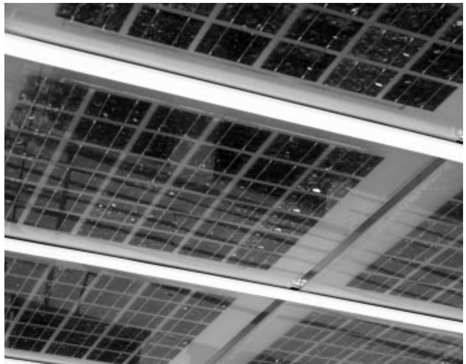
Figure 11. PV integrated into a skylight system at the Thoreau Center for Sustainability at Presidio National Park in San Francisco.
