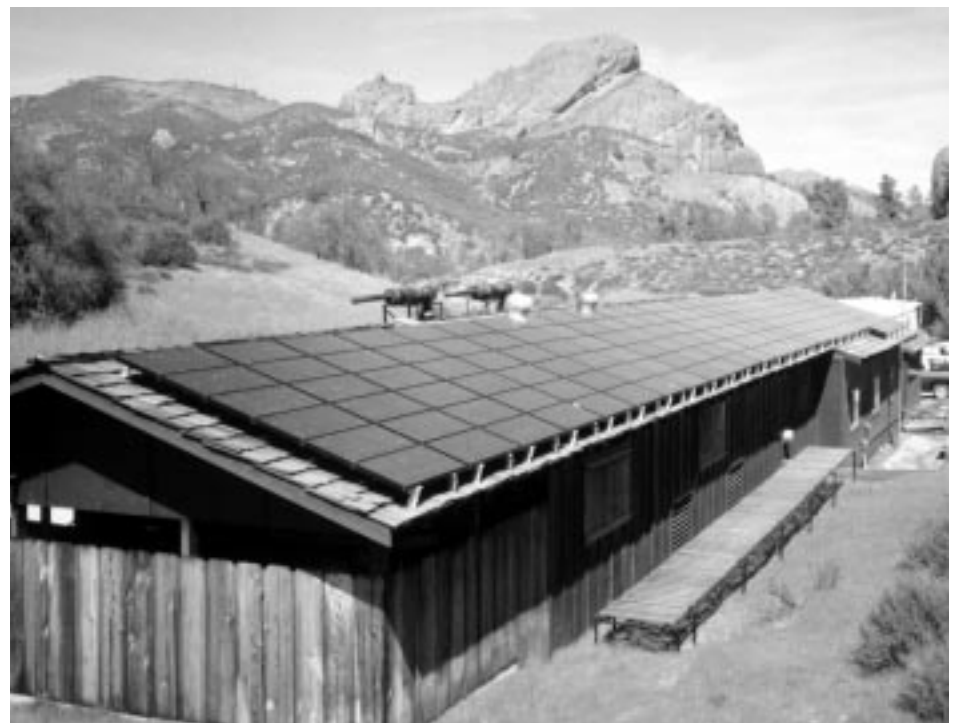
Figure 9. The PV array mounted on the roof of the maintenance building at Pinnacles National Monument.
