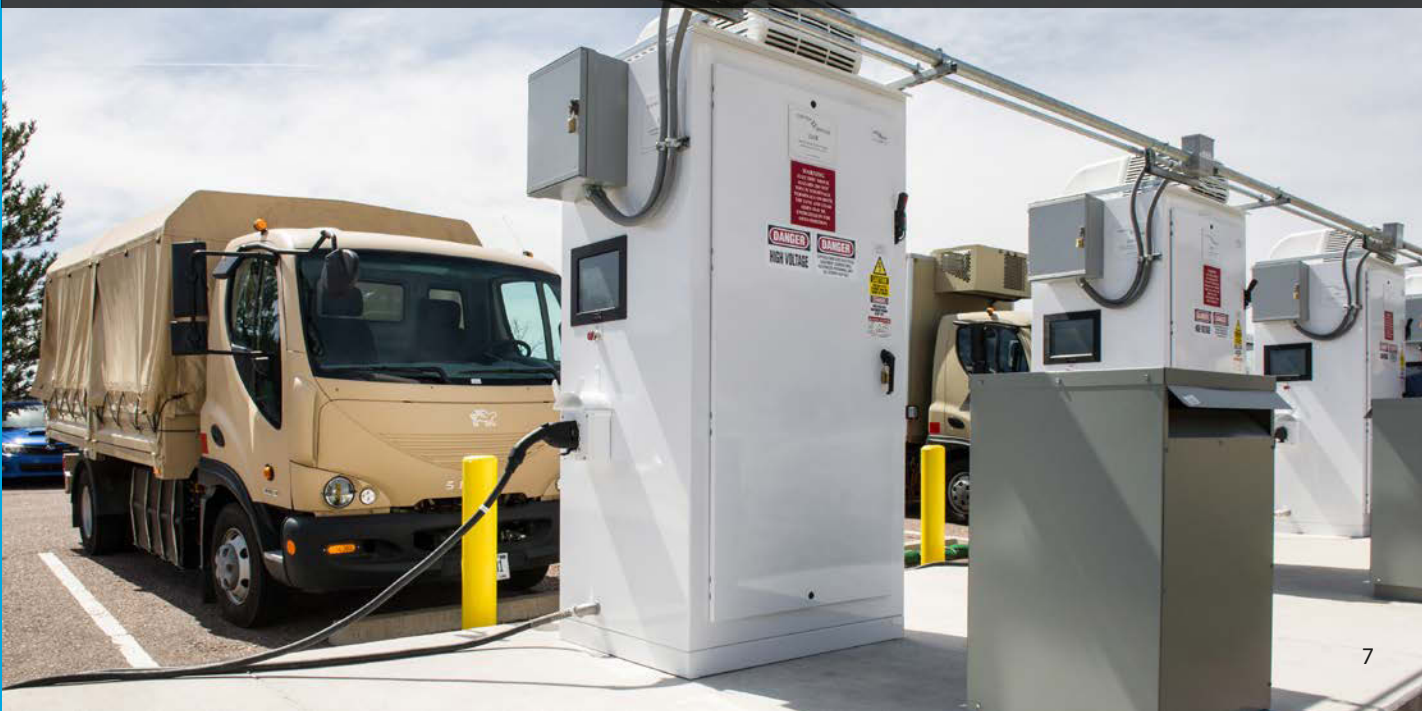
Army bi-directional electric vehicles docked at the Electrification Pilot Site at Fort Carson Army Base in Colorado Springs.
