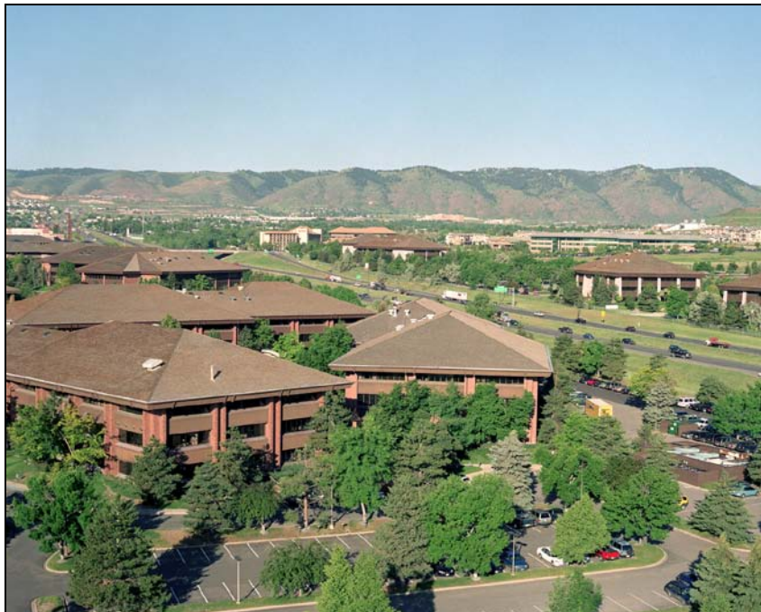
Figure 8. South Table Mountain site – Denver West Office Park
