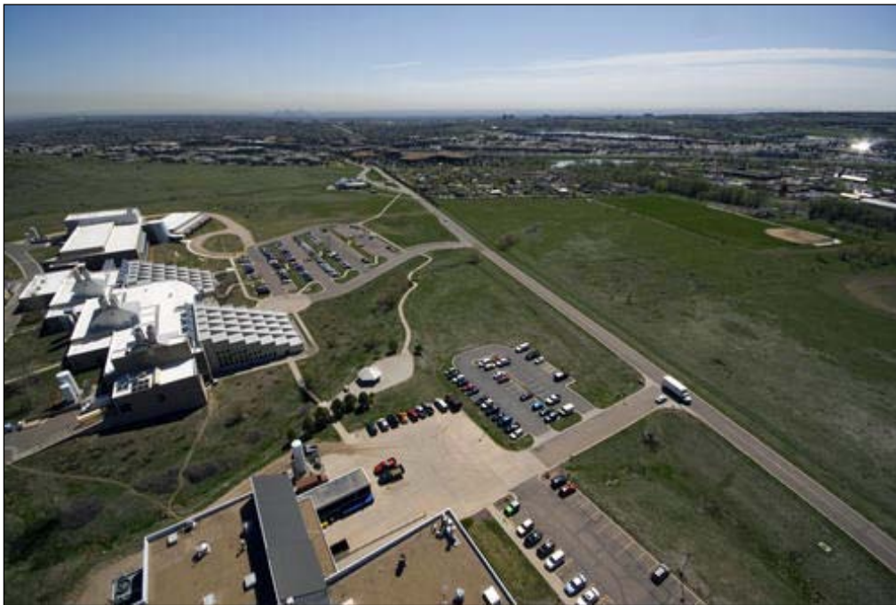
Figure 6. South Table Mountain site – east view
