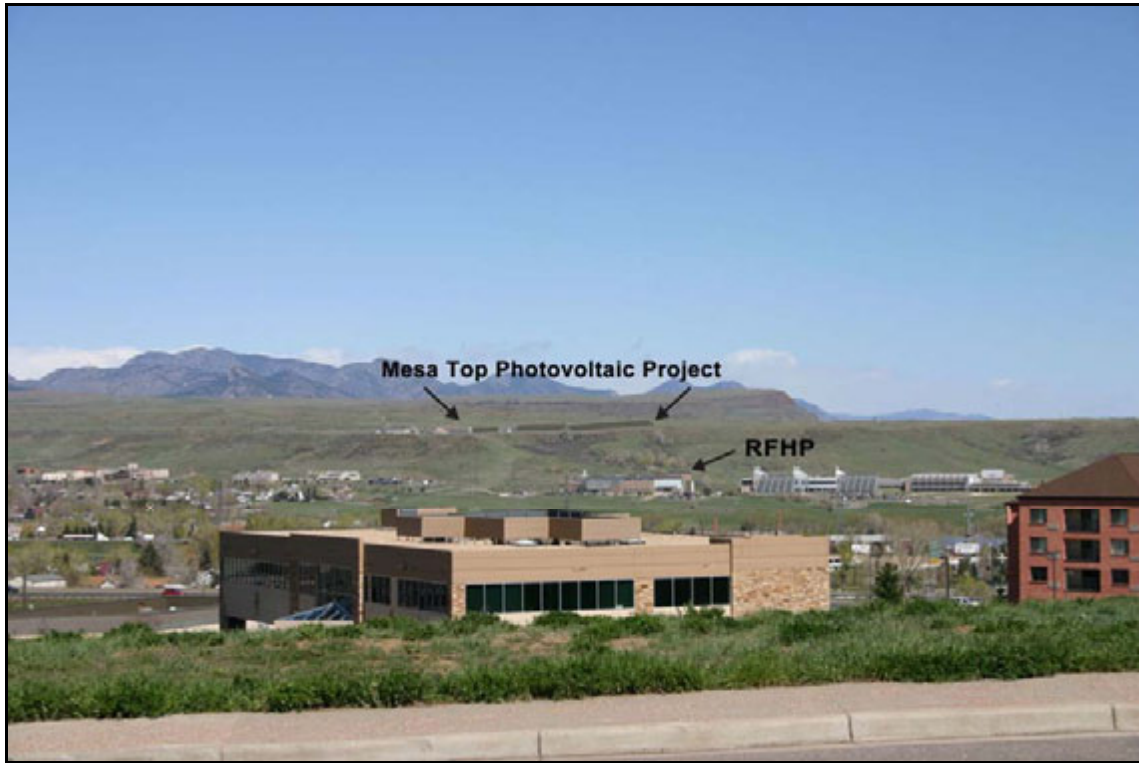
Figure 3-4. Simulated View of the Proposed RFHP, with the Proposed MTPP in the Distance
