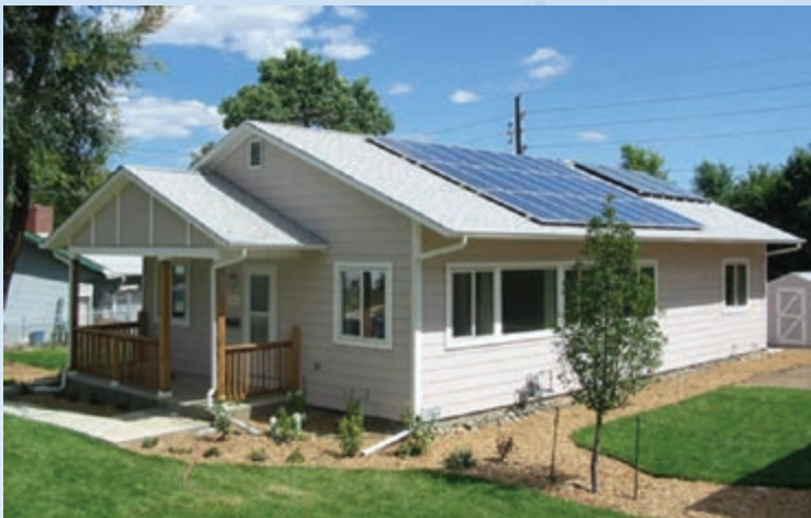
NREL and DOE-GO volunteers helped construct Denver's first net zero energy Habitat for Humanity home. Construction of this home was made possible through the sponsorship of the Laboratory's managing partners, MRI and Battelle.
