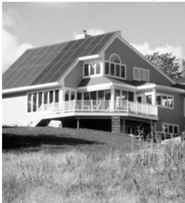
This house in coastal Maine generates its own electricity from a 4.25 kW PV system. Through a net-metering relationship with Central Maine Power, surplus solar electricity is exported to the utility grid, effectively spinning the utility meter backward. The owners get this power back in an even exchange at night, and during periods of low sun.
