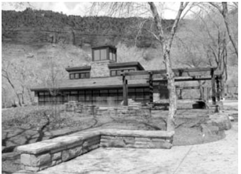
The National Park Service and NREL worked together to create this energy-efficient complex, the 7,600-square-foot Zion National Park Visitor Center. The building includes a 1,100-square-foot comfort station featuring daylighting, Trombe walls for passive solar heating, downdraft cooltowers for natural ventilation cooling, energy efficient lighting, and advanced building controls. These features are expected to result in energy cost savings of about $16,000 per year.
