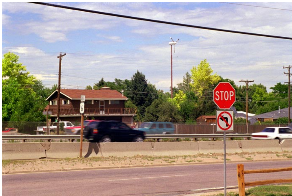
Figure 6. Enertech 1800 wind turbine from across the 6 th Avenue freeway, Lakewood, Colorado, Case Study 6.
