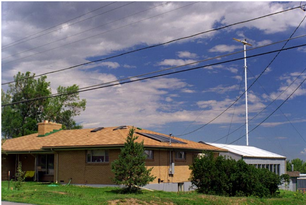
Figure 5. WhirlWind 4000 wind turbine behind home with solar hot-water panels, Jefferson County Colorado, Case Study 5.
