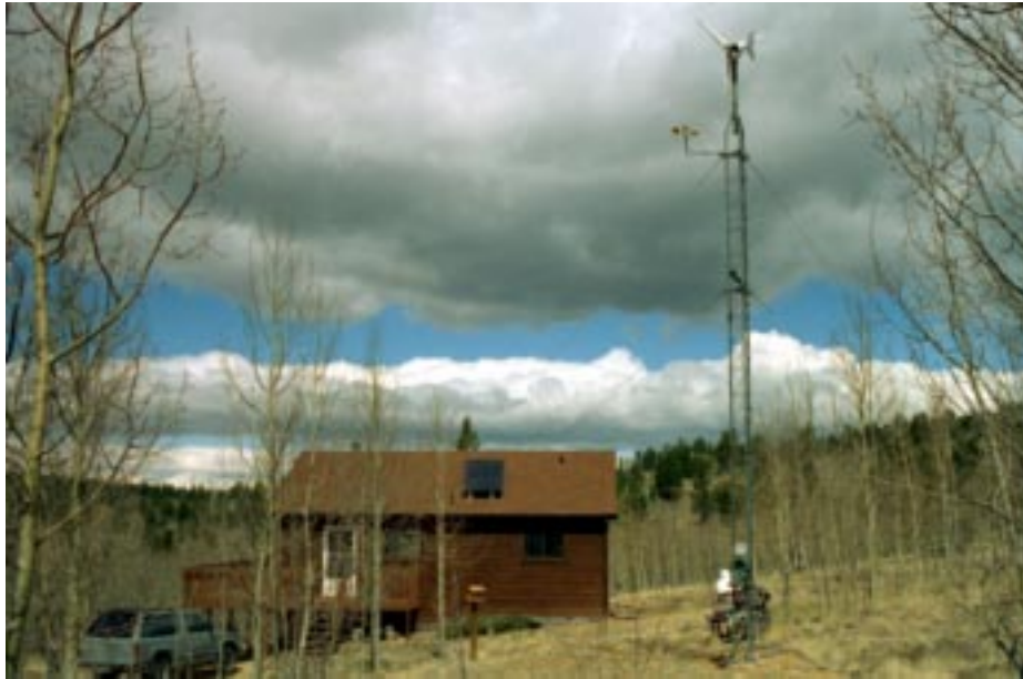
Figure 3. Southwest Windpower 503 adjacent to South Park mountain cabin with PV panels on roof, Case Study 3.
