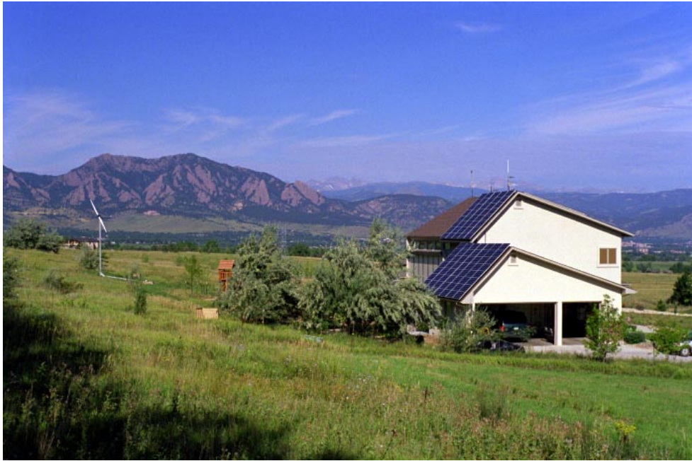
Figure 2. Whisper 3000 wind turbine adjacent to passive-solar home with PV panels on roof, Case Study 2.
