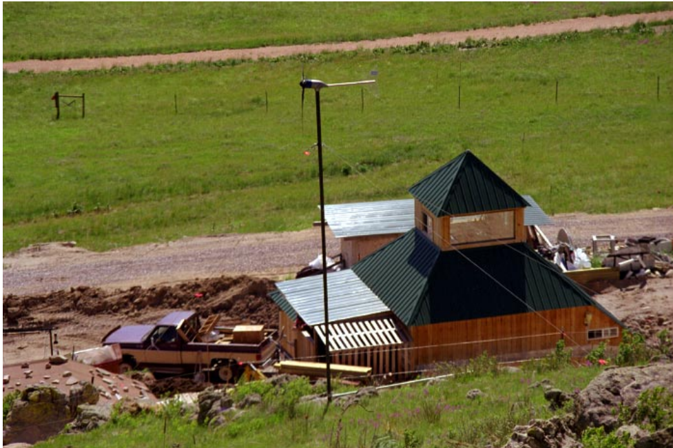
Figure 1. Whisper 900 wind turbine on hillside above Douglas County home, Case Study 1.
