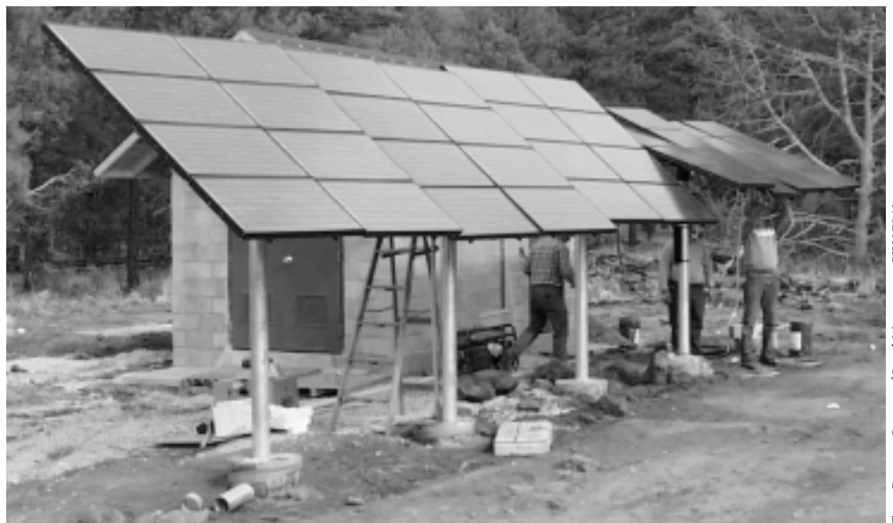
Array installation at Mt. Trumbull; the power center, inverters, batteries, and generator are located in the nearby building.
