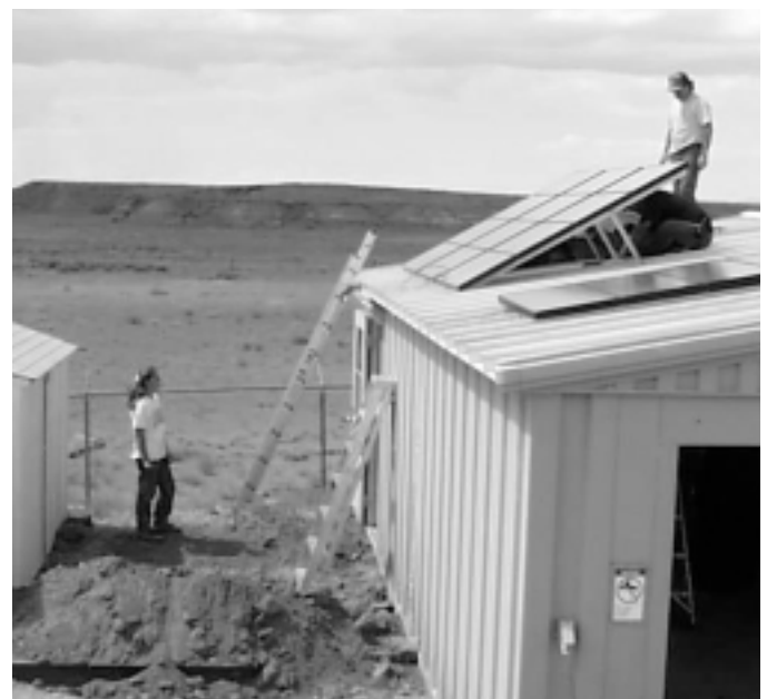
A PV array is installed on the roof of a garage at Parriette Field Station in Utah.
