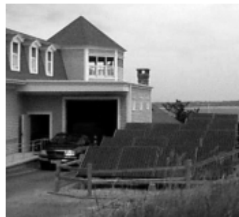
The Block Island Post Office PV system
