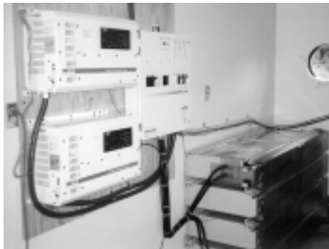
The power center, inverter and battery installation at Chimney Peak are typical of those at all five facilities.
