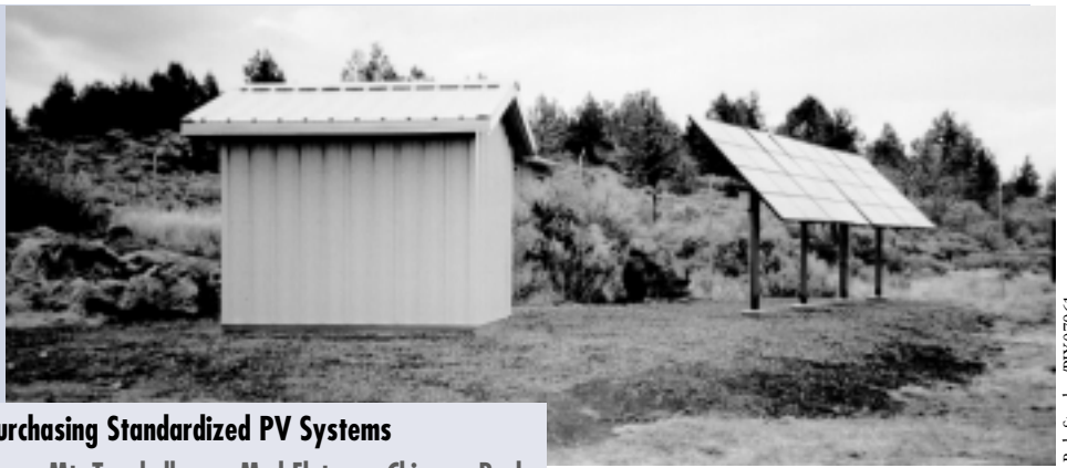
Batteries and controls are located inside this steel building at Mud Flat Station in Idaho.
