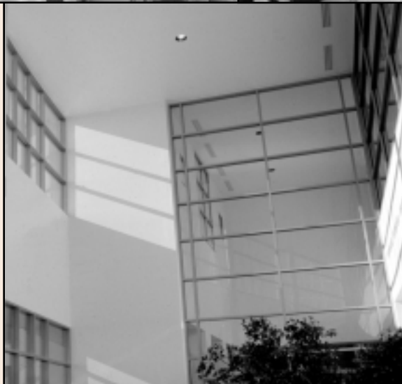
Warren Gretz, NREL/PIX02193
