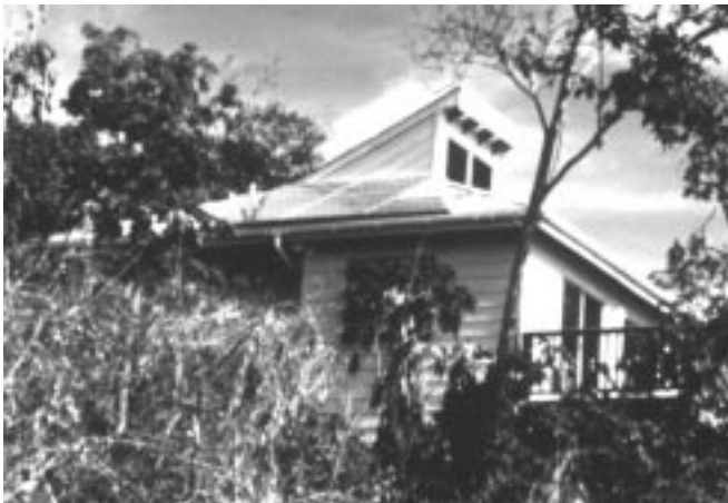
Figure 3. One of the vacation cabins at Harmony Resort on the Island of St. John in the Virgin Islands. The PV unit, which survived Hurricane Marilyn without damage, can be seen on the roof (photo by John Thornton, NREL).
