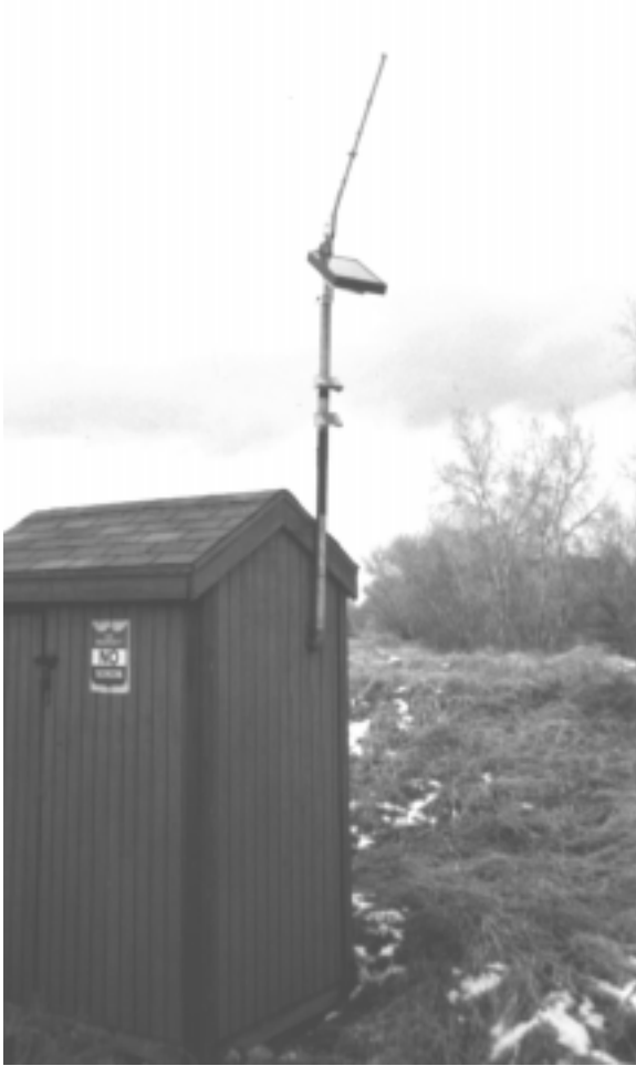
Figure 1. A PV-powered water-level monitor protects the City of Ft. Collins, Colorado, from floods by continually monitoring stream flow and radioing data to the city center. Alarms are triggered if the stream rises to dangerous levels, and emergency response procedures are started (photo by John Thornton, NREL).
