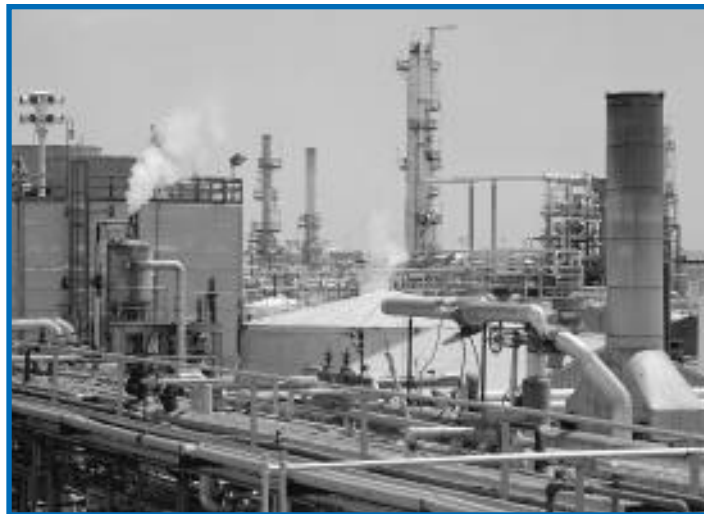
Review of a refinery's boiler, steam distribution, and condensate systems revealed potential energy savings of $1 million+.
