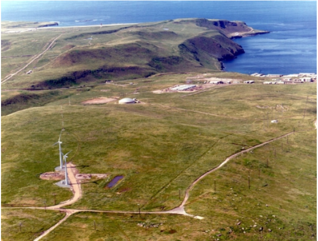
Figure 8: SCI Naval Facilities and SERDP Wind Farm Site Source: USN NFESC Aerial Photograph
