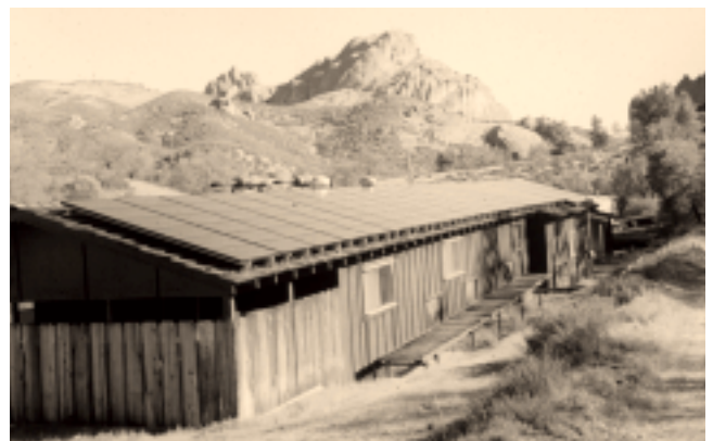
This quiet, unobtrusive hybrid photovoltaic system provides the Chapparral area on the west side of Pinnacles National Monument with clean, reliable electricity. In this pristine area, the photovoltaic installation eliminates park service staff concerns about fuel spills or leaks, because the PV system requires no fuel and produces no emissions.
