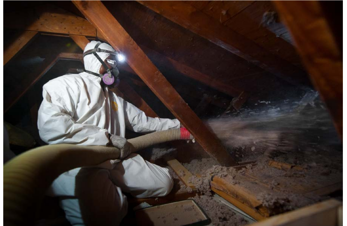
Insulation blown into an attic. Photo by Dennis Schroeder, NREL 17956
