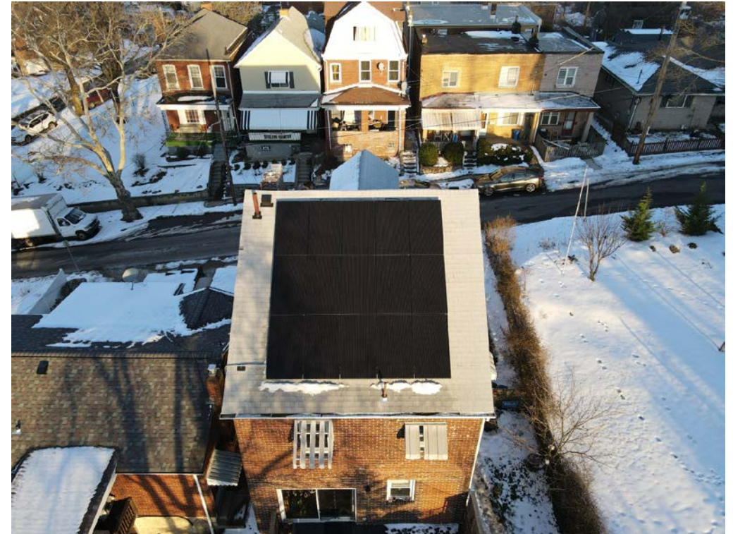
Solar PV in Pittsburgh. NREL Image 66338
