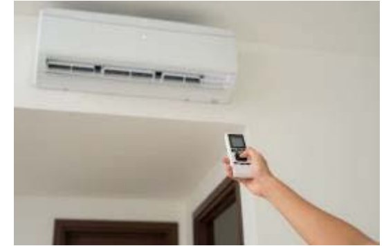
Mini-split heat pump inside head unit. Image from Building America Solution Center
