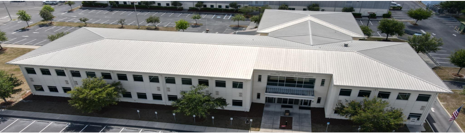
The Brandon Support Operations Complex (BSOC) in Hillsborough County. [Credit: Hillsborough County]
