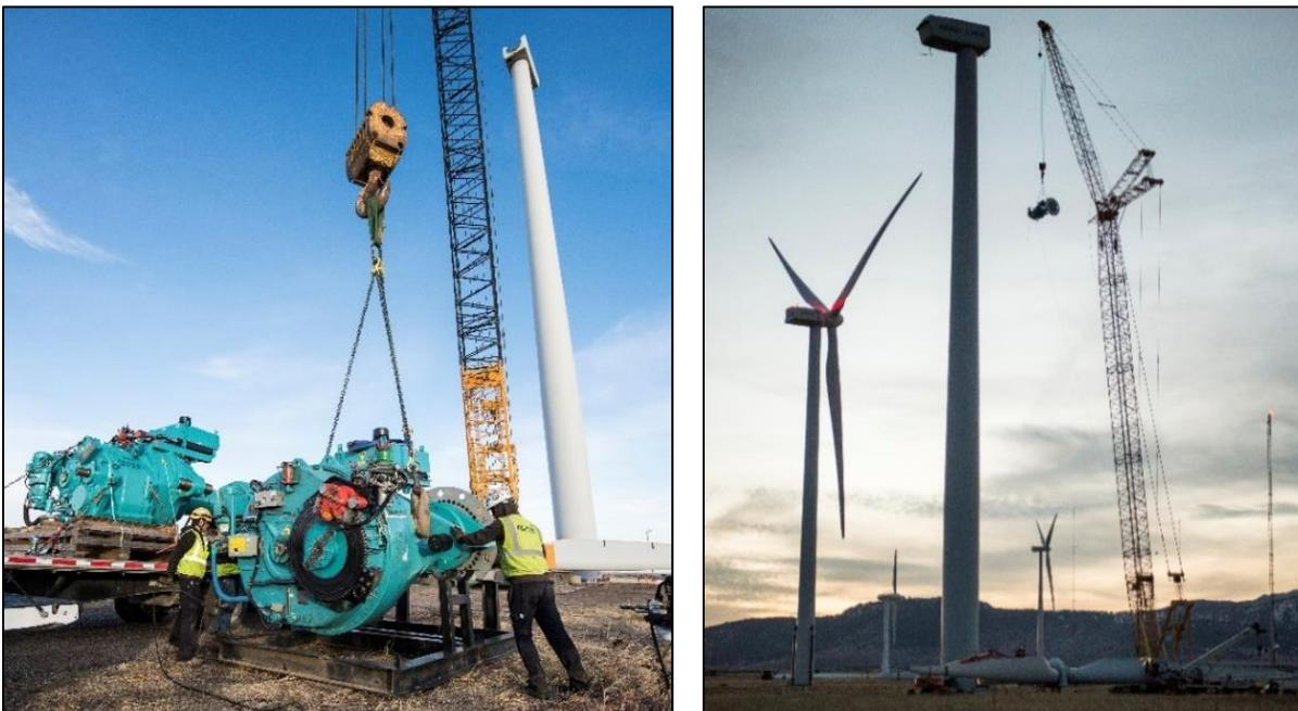
**Figure 8. Gearbox swap (left) and installation in turbine (right). Photos by Dennis Schroeder, NREL 49409 and 49413**
