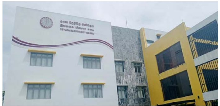
The front office of the Ceylon Electricity Board's national system control centre. Photo courtesy of Thushara de Silva, NREL.
