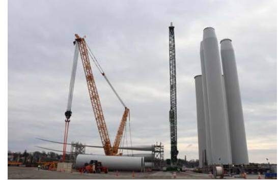
Components await transport to the South Fork Wind project at State Pier in New London, Connecticut. Photo by Matilda Kreider, NREL
