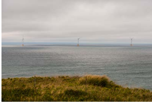
Some of the turbines in the Block Island Wind Farm. Photo by Dennis Schroeder, NREL 40473
