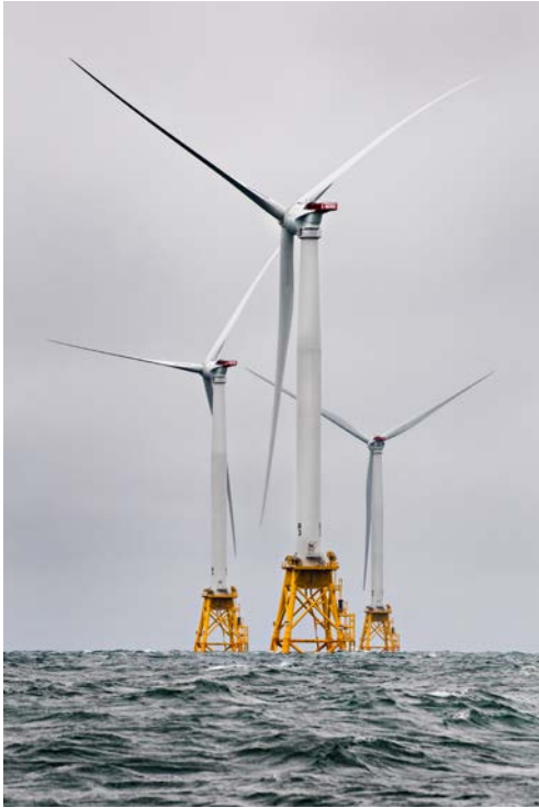
Photo by Dennis Schroeder, NREL 40484
